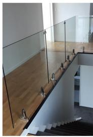
• MP10 has a fixed clamping plate with oval base and suits 12mm toughened safety glass only.
